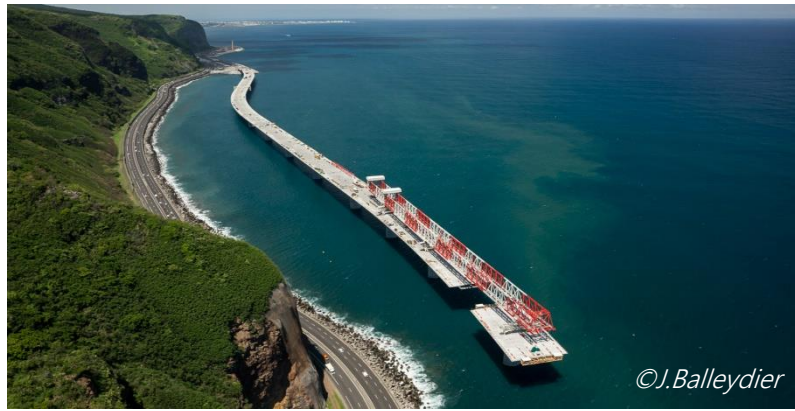
New water front road
