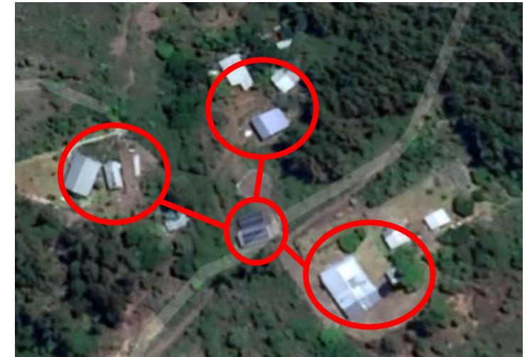
Figure 6 – Satellite picture of the solar powered microgrid
